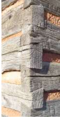
Notch and Chamfer Dovetailing
