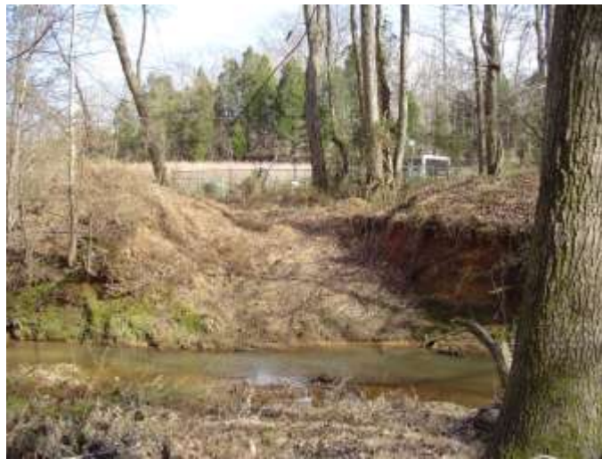
Embankment cut on Clems Branch. Possible historical road crossing. View south over creek to campground in the distance.
